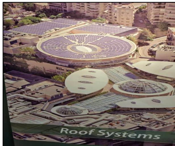
Fig. 2. Solar PV panels on the roof of terminals and administration buildings
