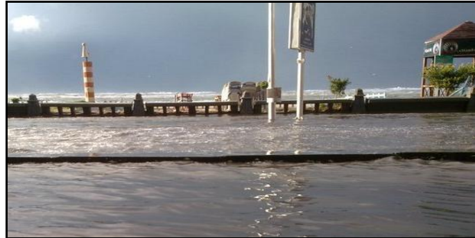
Figure 5. Wave flooding due the sea level rise at Alexandria coastline, 2010.
