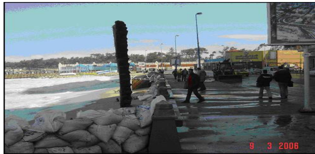
Figure 2. Erosion and flooding occurring at Alexandrian coastline.
