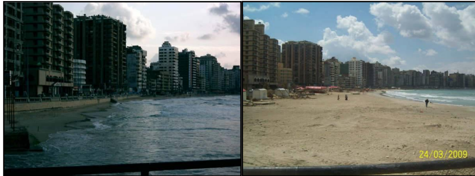
Figure 18: Comparison between the beach width after and before the construction of the submerged breakwater at Mandra beach (El-Sharnouby & Soliman, 2010)
