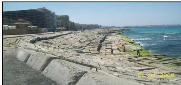
Figure 9: Reinforcement of beach profile by concrete revetment at Loran.
