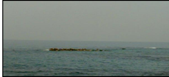
Figure 14: Failure of the detached breakwater at Cleopatra beach.
