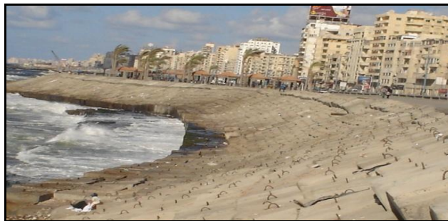
Figure 7: Shore protection by concrete cubic blocks at Sporting beach.
