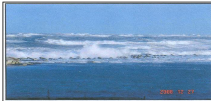
Figure 13: Efficiency of the submerged breakwater at 7.0 meter depth in storm time.
