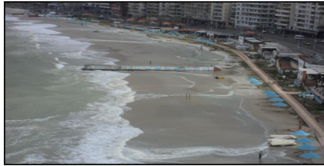
Figure 20: Effect of submerged breakwater in the protection of Miami beach during the storm of winter 2010.
